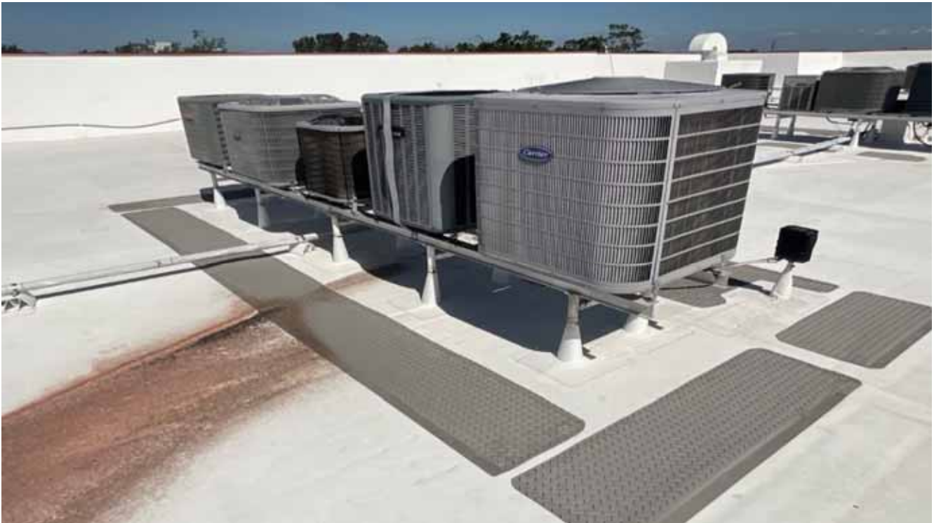
South Condo Bldg Roof A/C Stand - Typical
