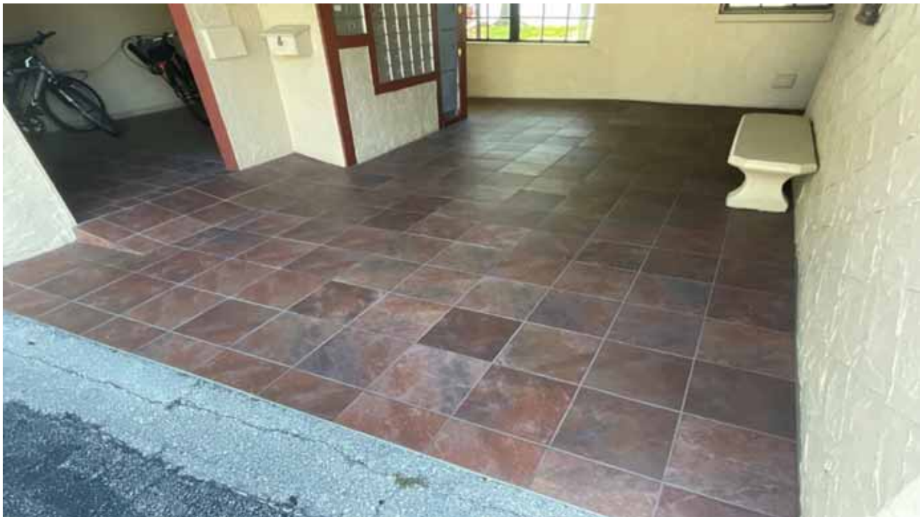
South Condo Bldg Lobby Tile
