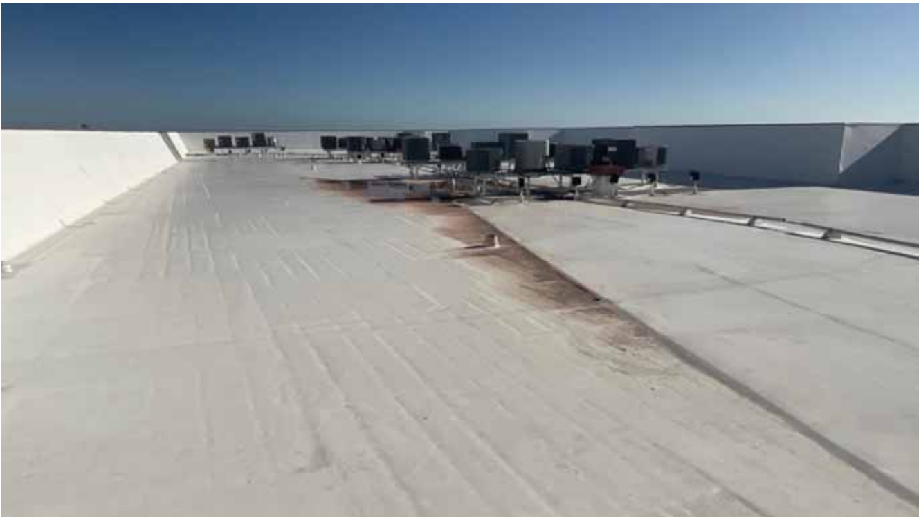
North Condo Bldg Roof
