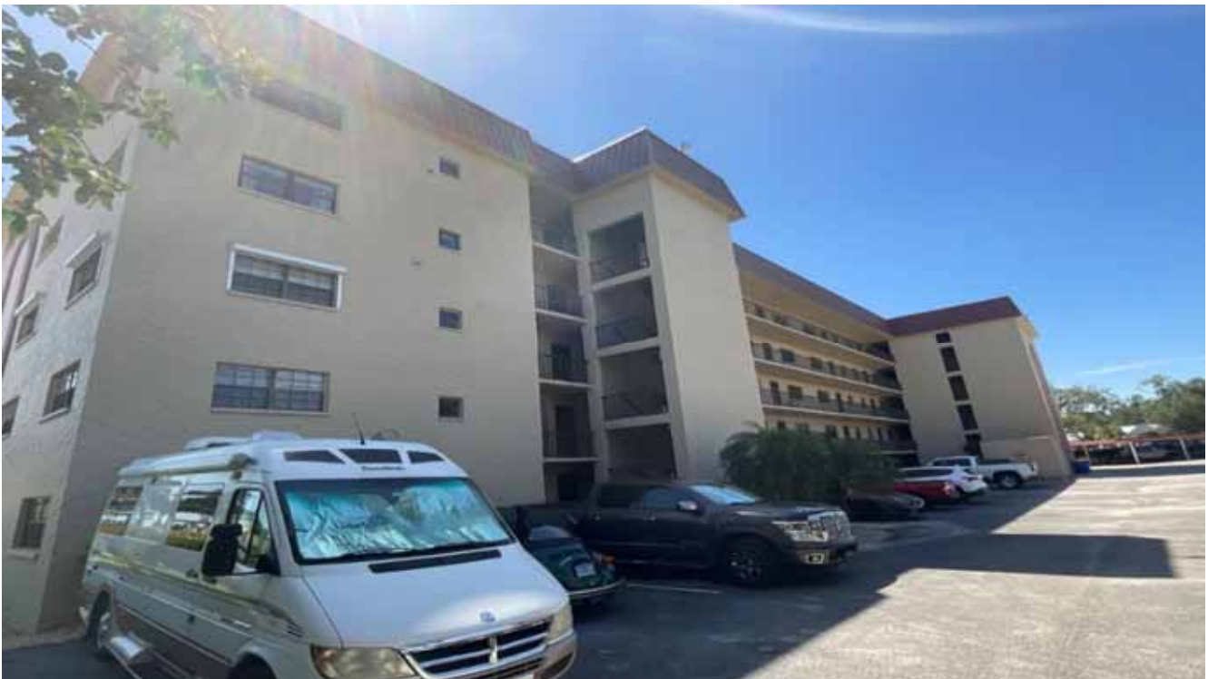
North Condo Bldg
