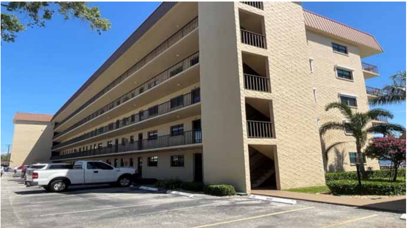
North Condo Bldg
