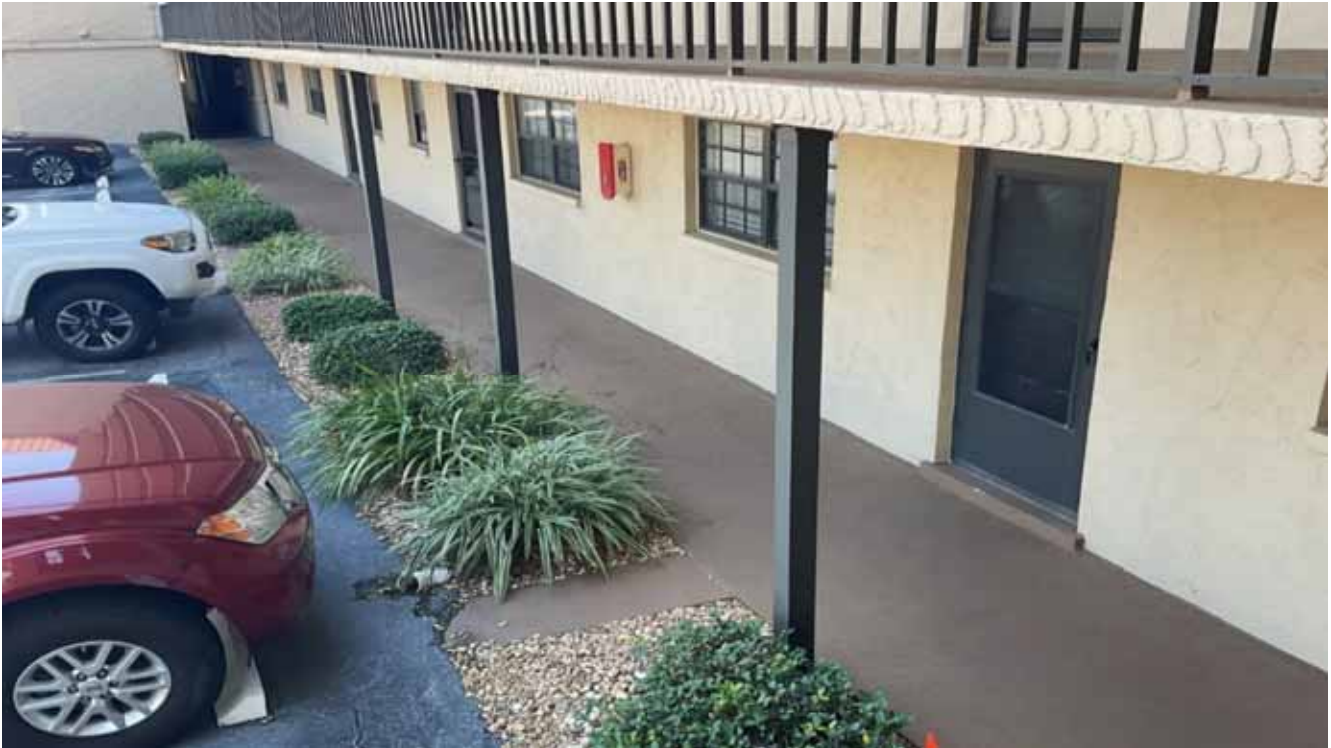
South Condo Bldg Support Posts
