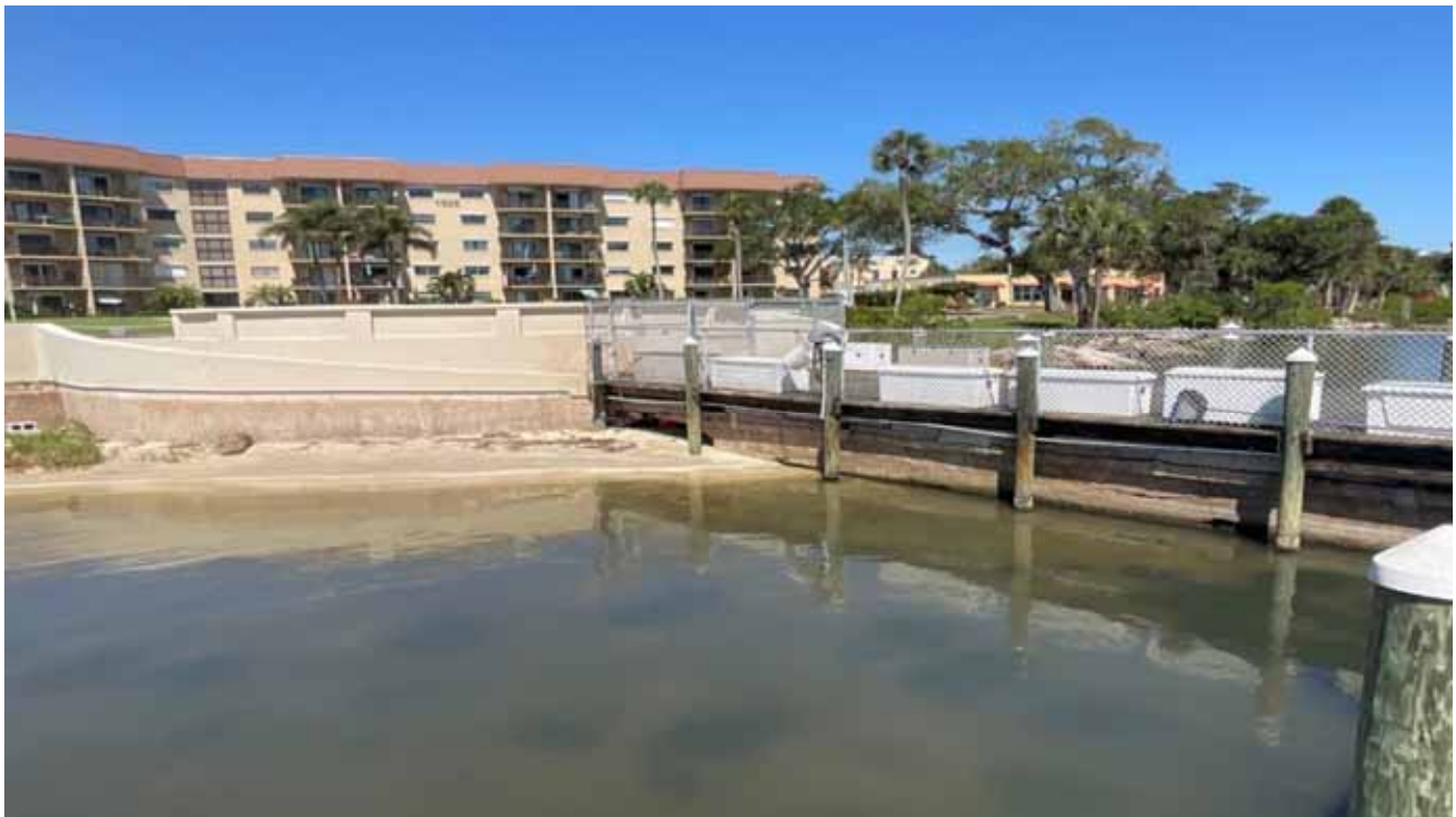
Seawall & Boat Dock
