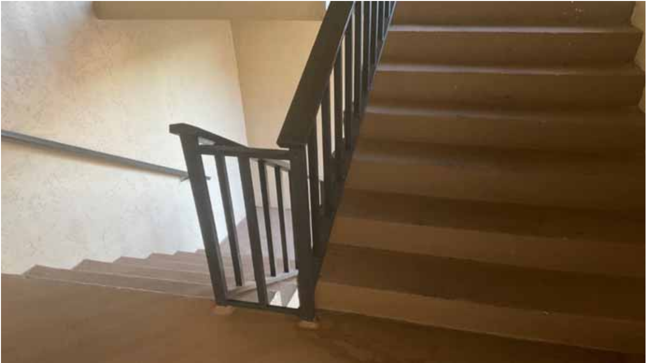
North Condo Bldg Stairwell
