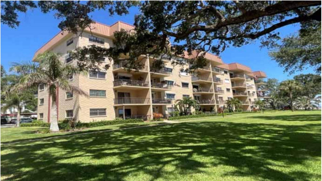
South Condo Bldg
