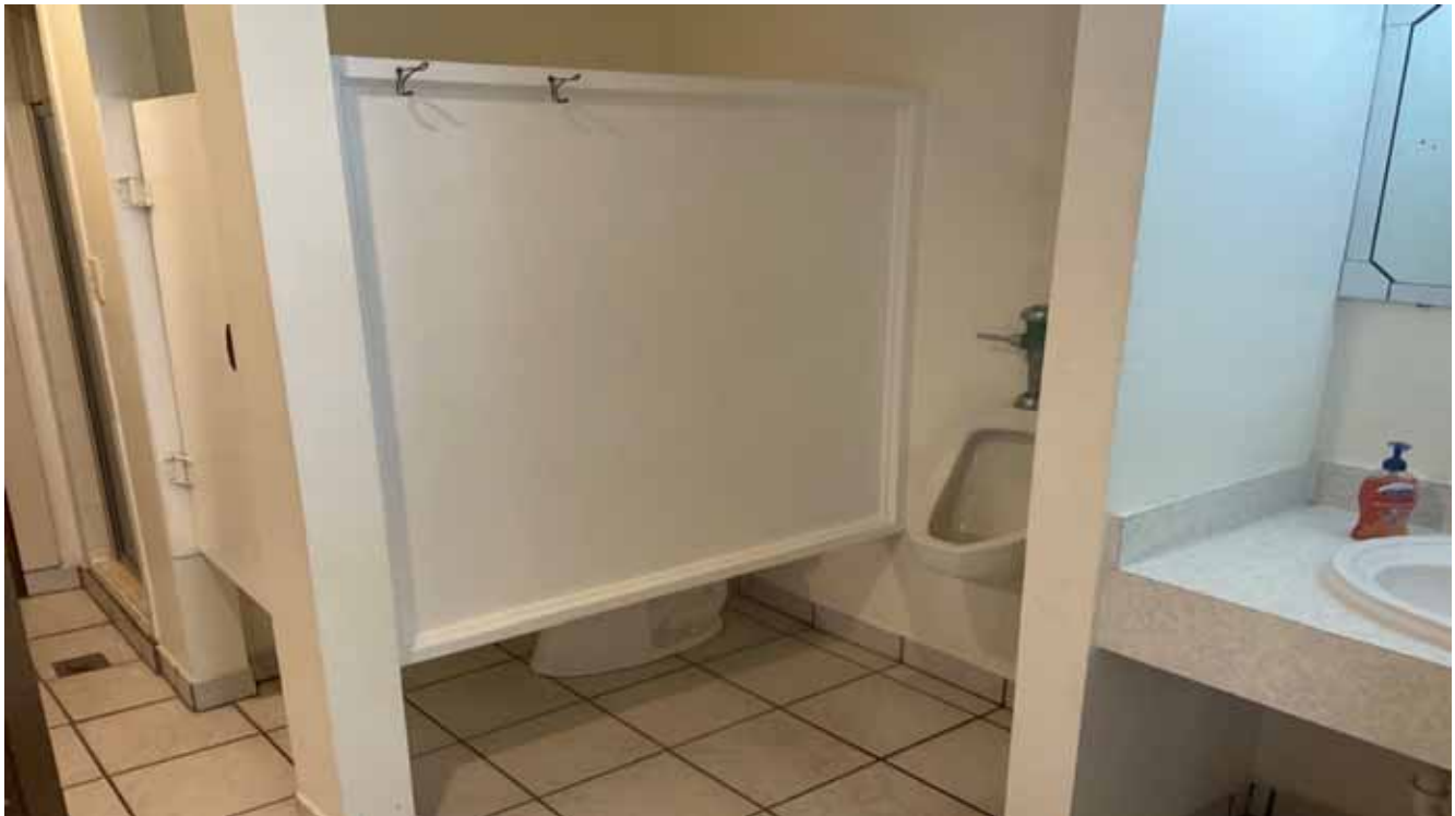
Pool House Bldg Restroom, Men's
