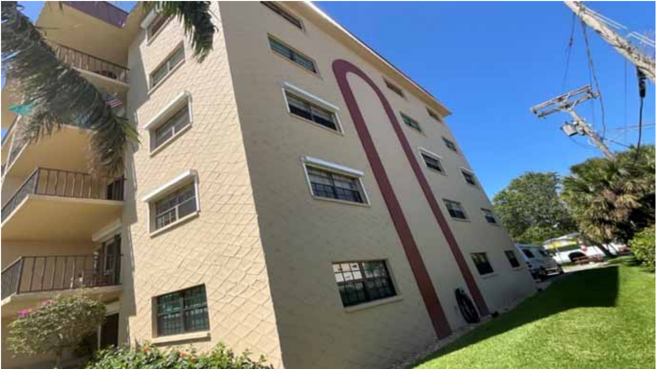
North Condo Bldg
