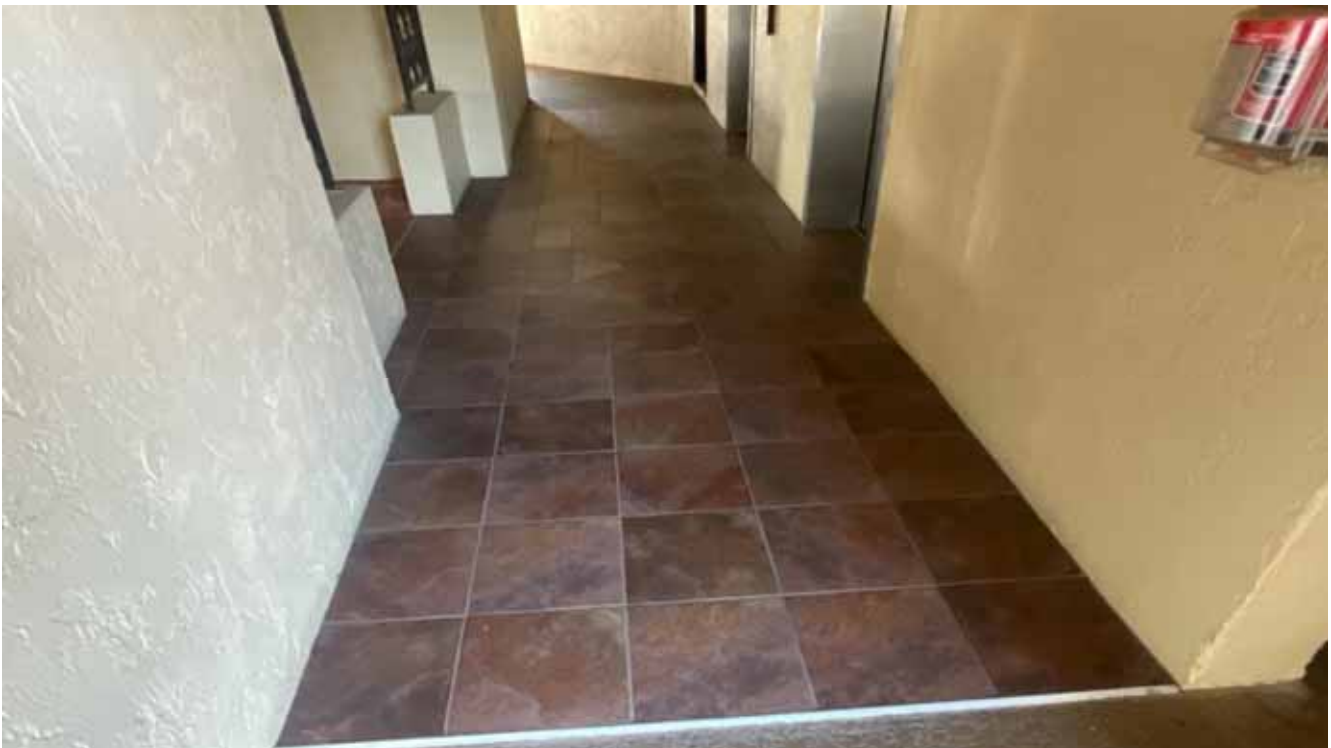
North Condo Bldg 1st Floor Tile
