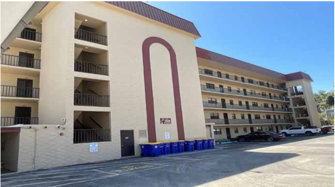
South Condo Bldg
