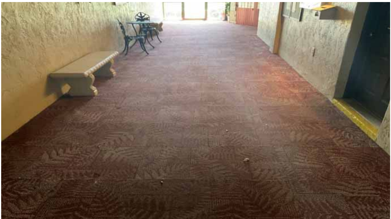
North Condo Bldg 1st Floor Carpet
