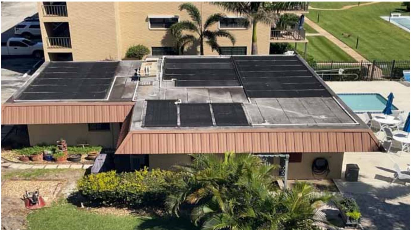
Pool House Bldg Roof & Pool Solar Panels
