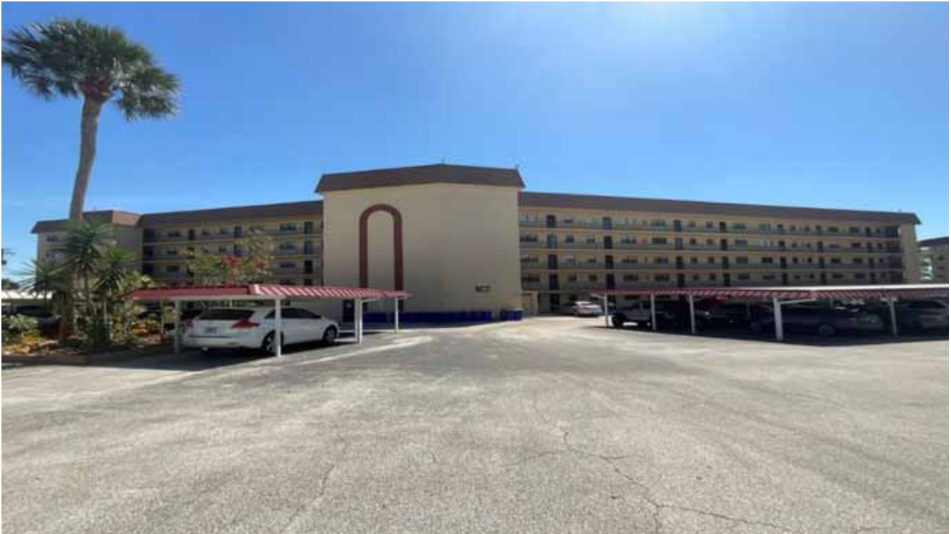
North Condo Bldg
