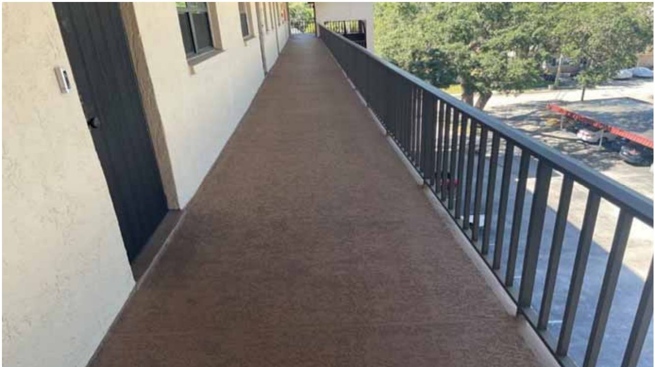
South Condo Bldg Common Walkway
