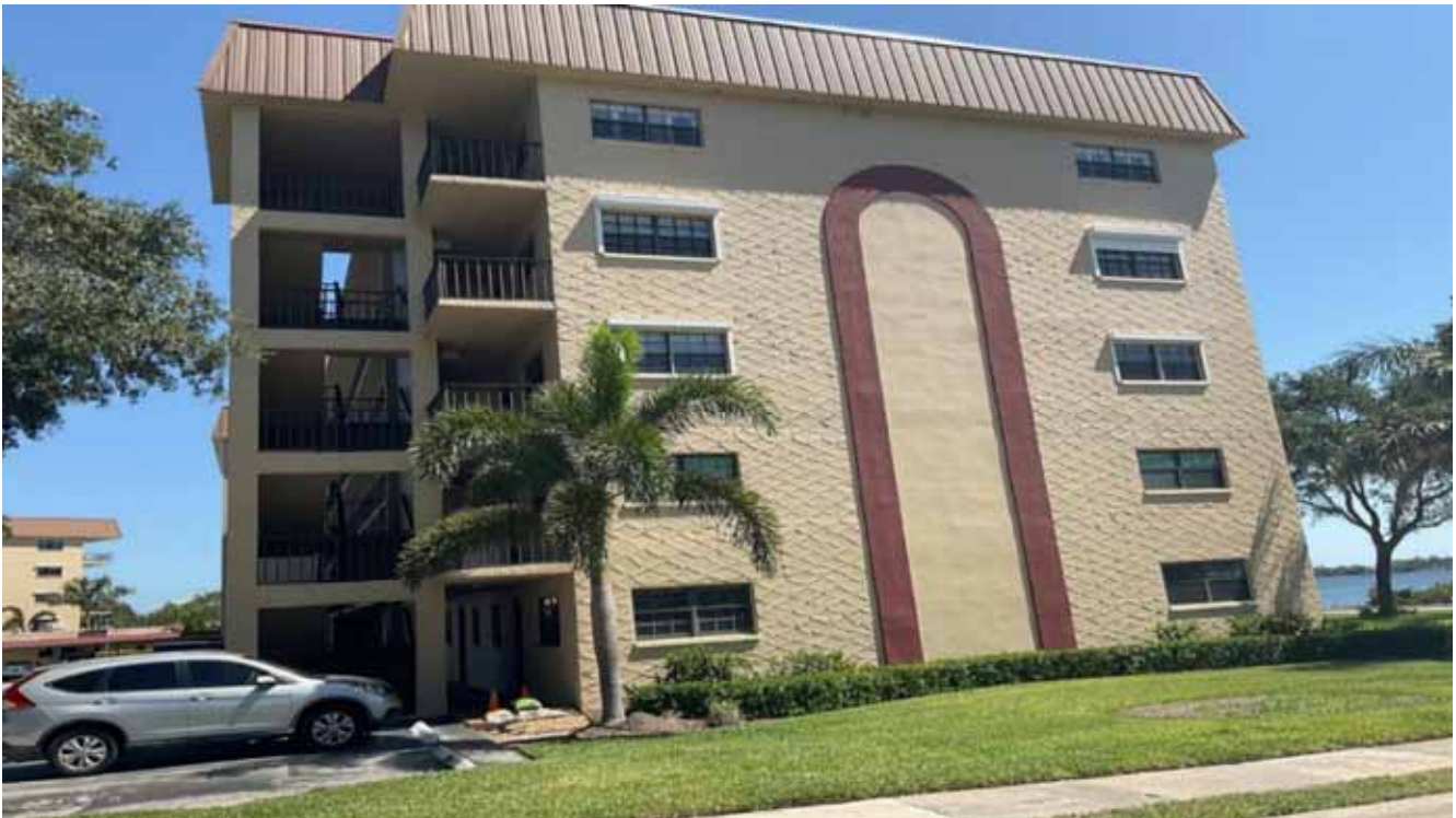
South Condo Bldg
