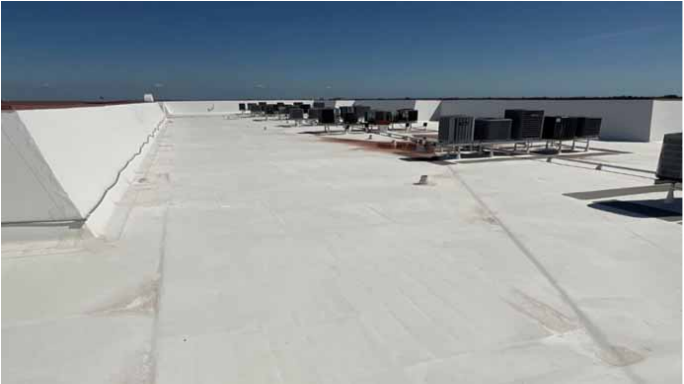
South Condo Bldg Roof
