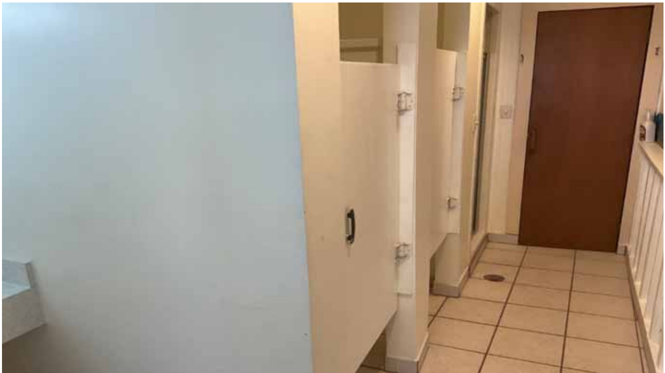
Pool House Bldg Restroom, Women's
