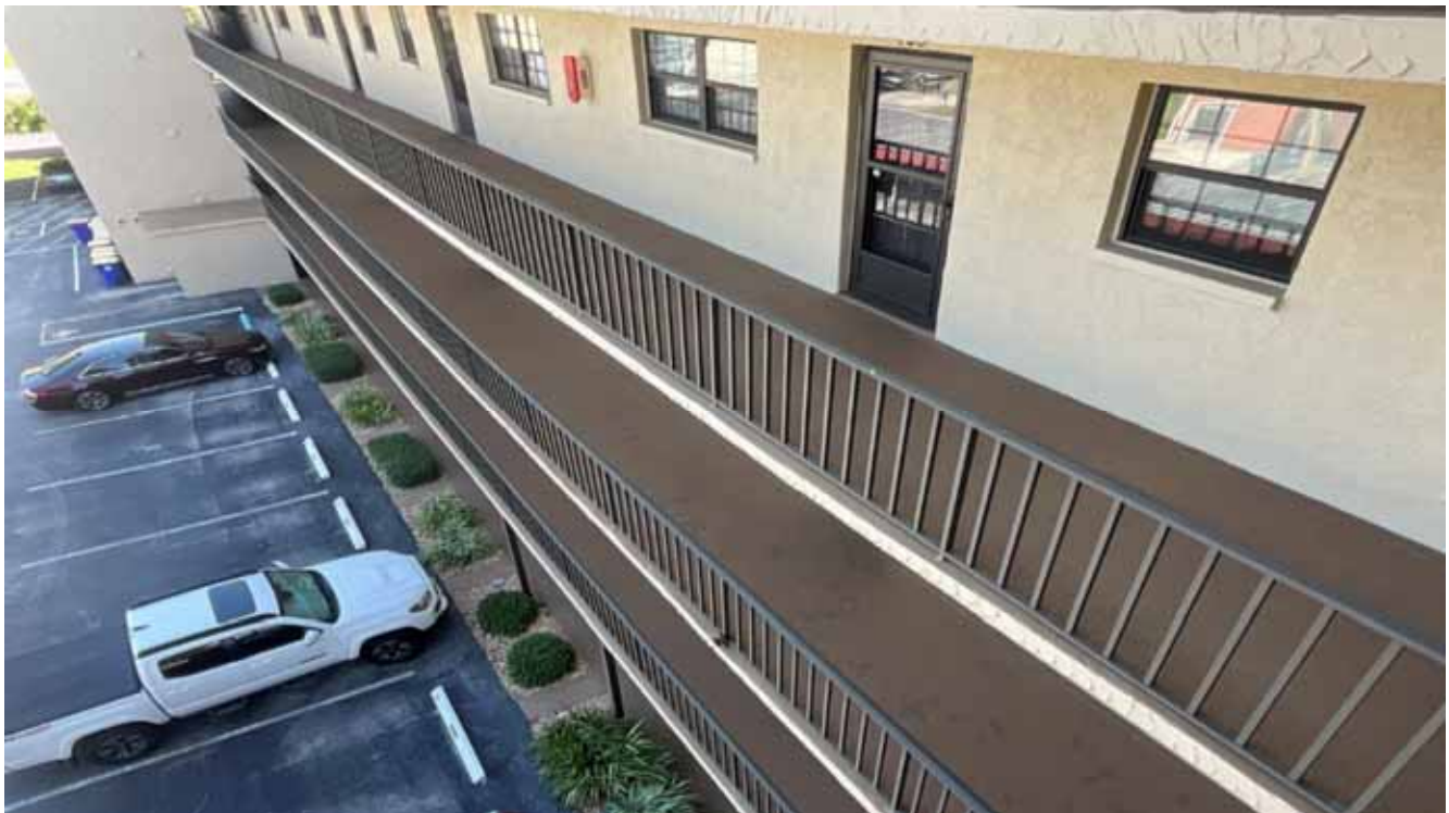
South Condo Bldg Common Walkways & Railing
