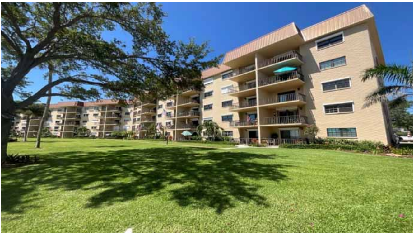
North Condo Bldg
