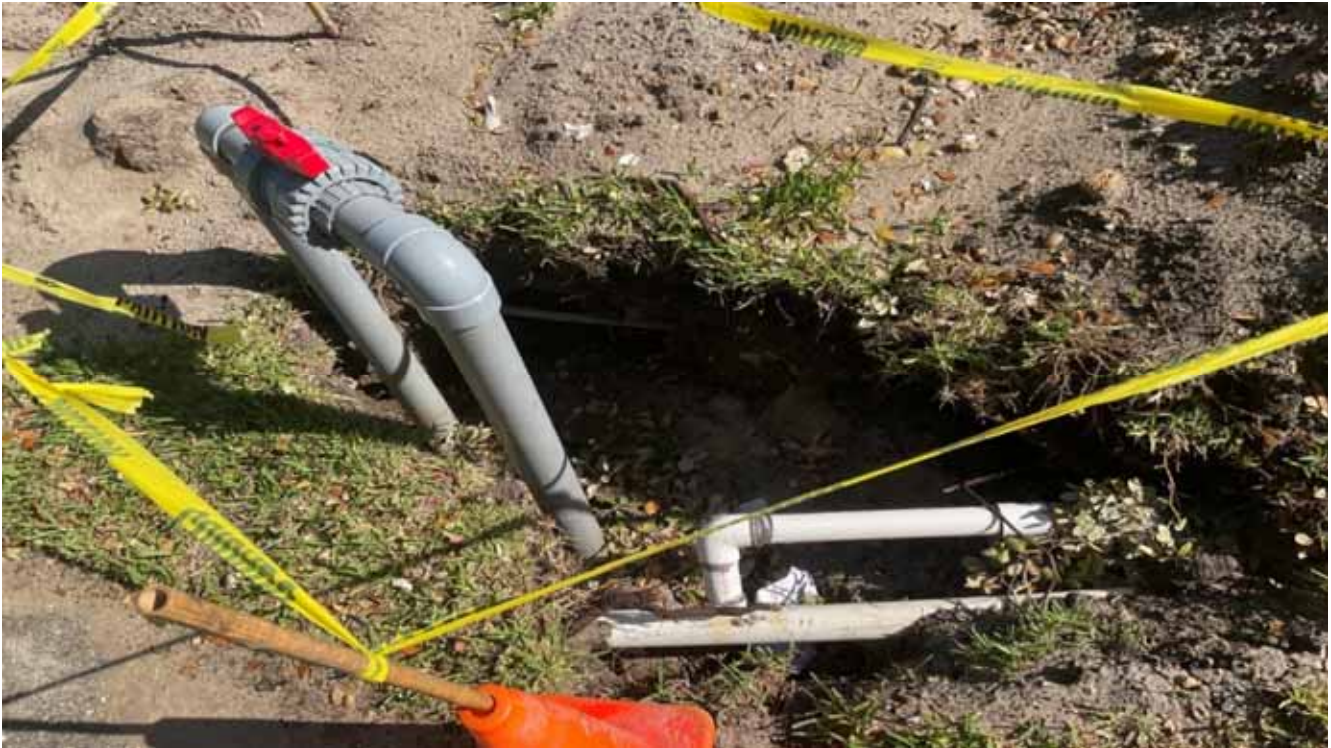
Fire Line Break
