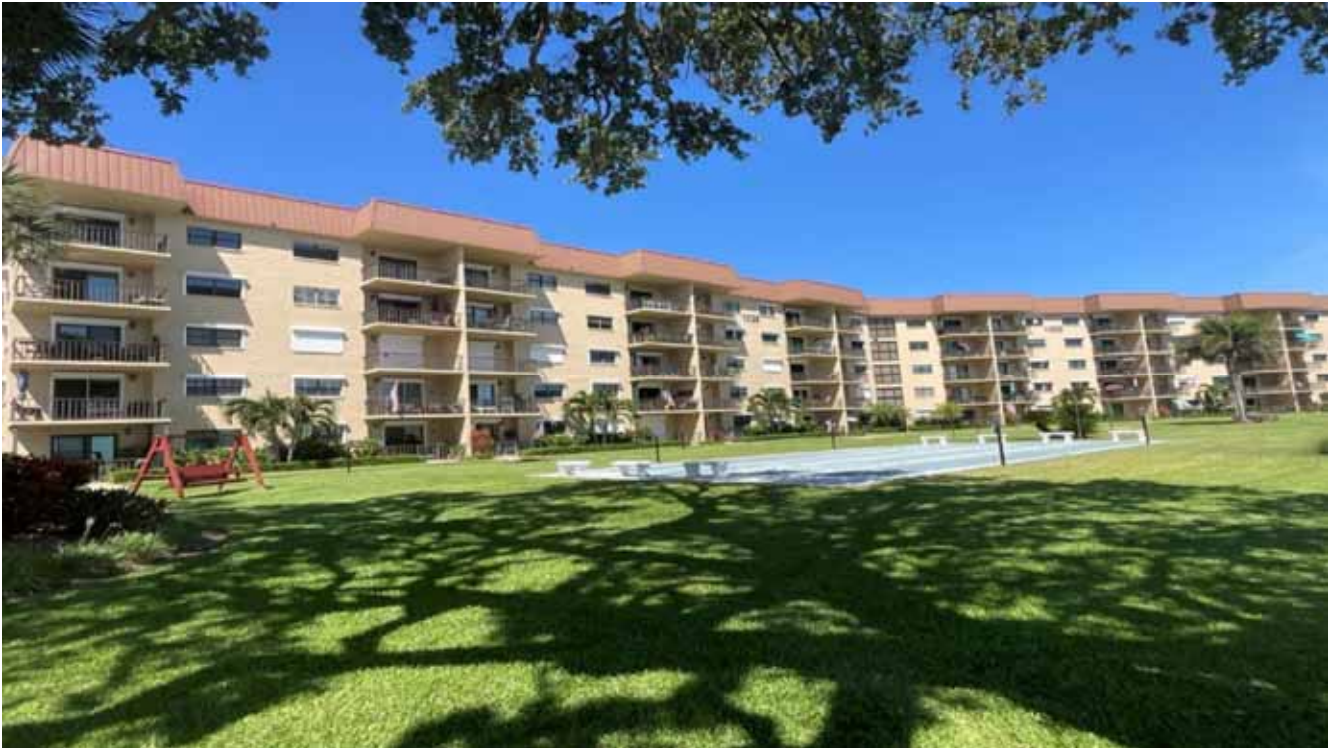
North Condo Bldg
