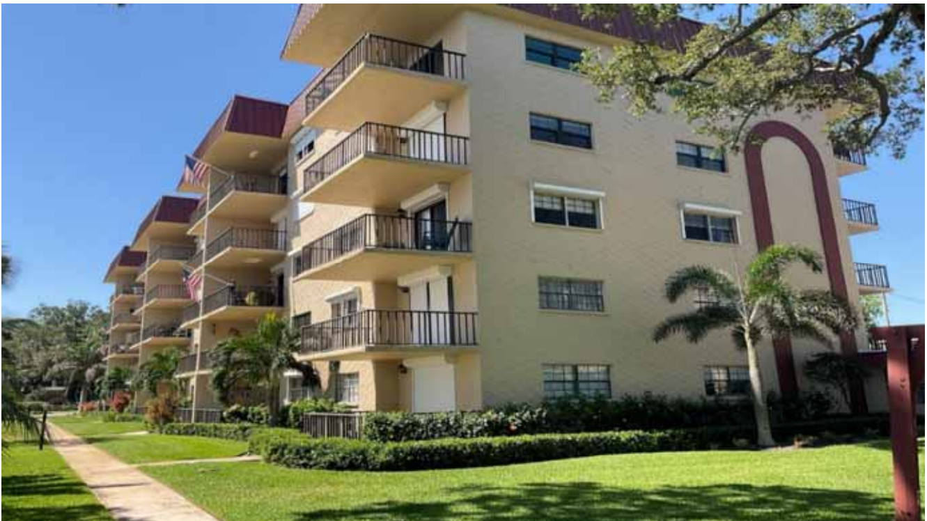
South Condo Bldg
