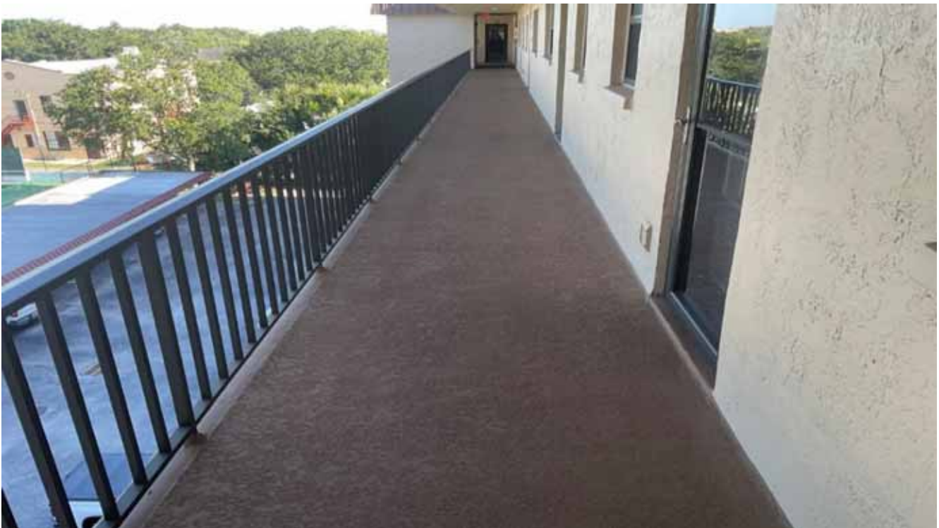
North Condo Bldg Common Walkway
