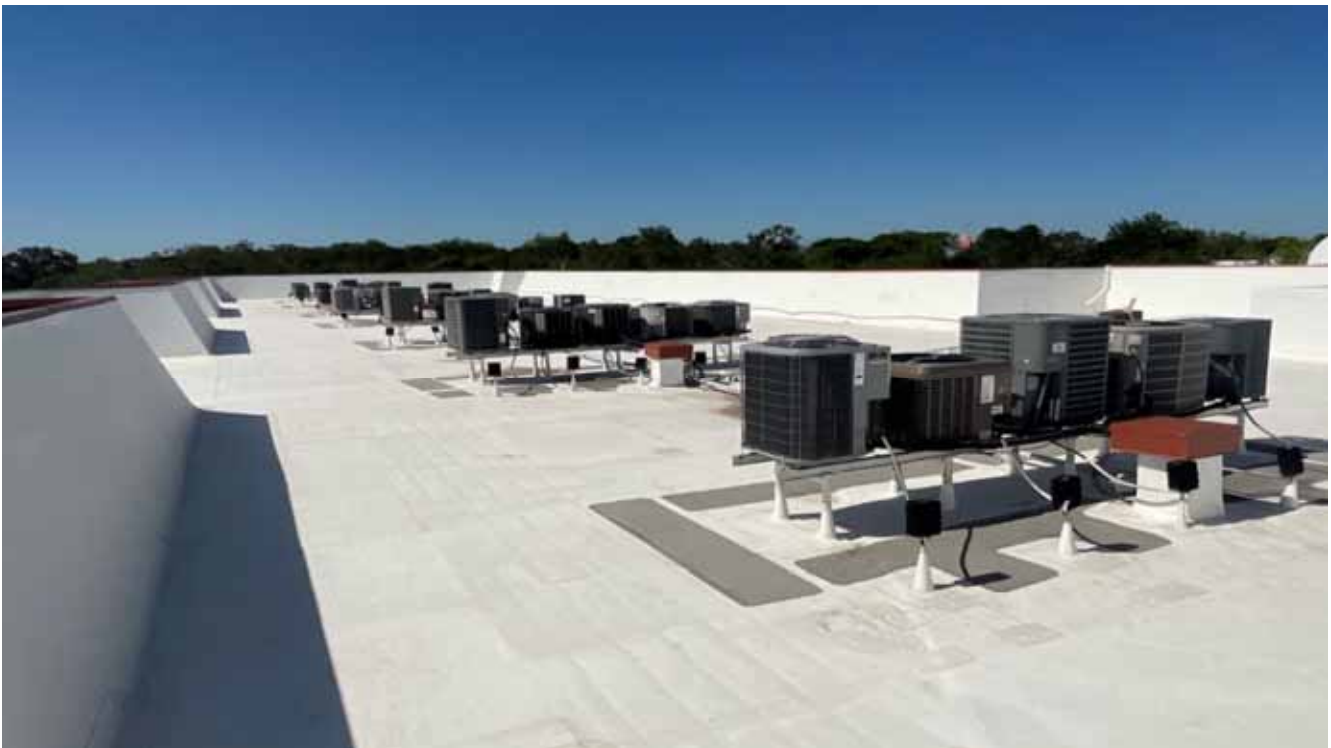
South Condo Bldg Roof
