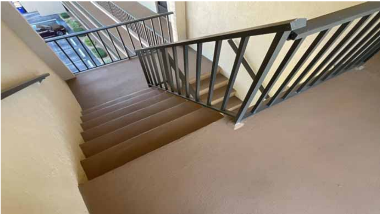
South Condo Bldg Stairwell
